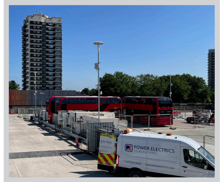
Henley Road: New garage build in progress.
